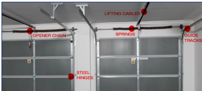
Figure 72: Garage Door Components
