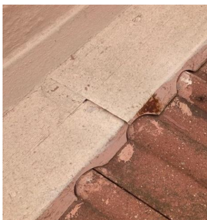
Figure 61: Failing Flashing
