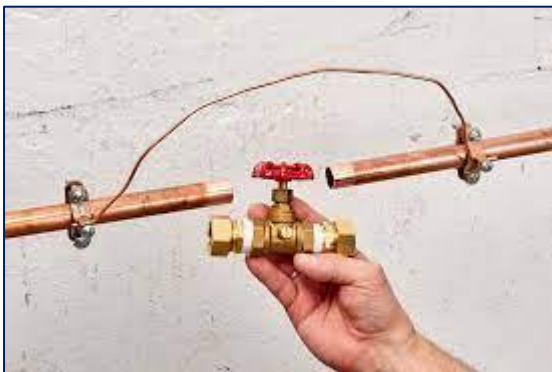
Figure 5: Main Water Shut-Off
