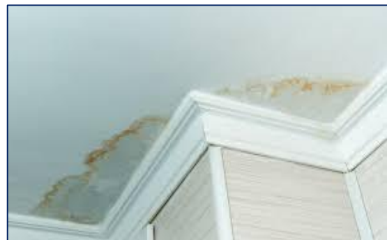
Figure 41: Water-Stained Ceiling
