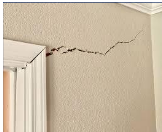
Figure 39: Structural Crack
