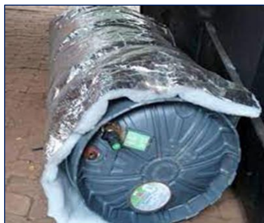
Figure 42: Insulated Geyser
