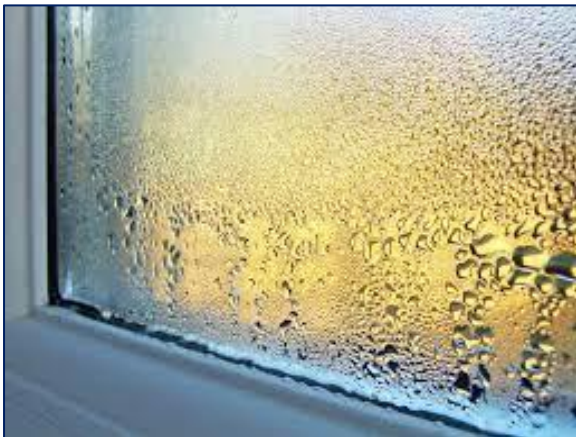
Figure 12: Condensation
