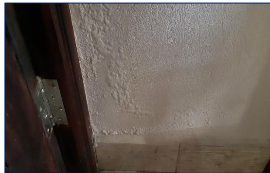
Figure 37: Moisture Intrusion
