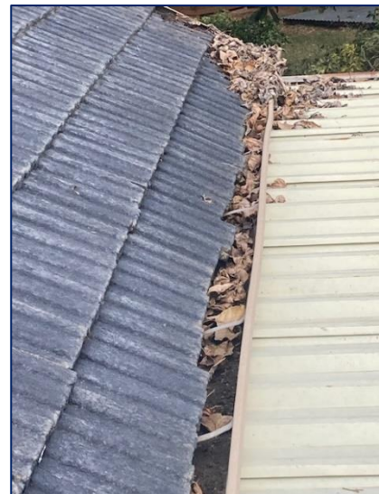
Figure 59: Clogged Gutter
