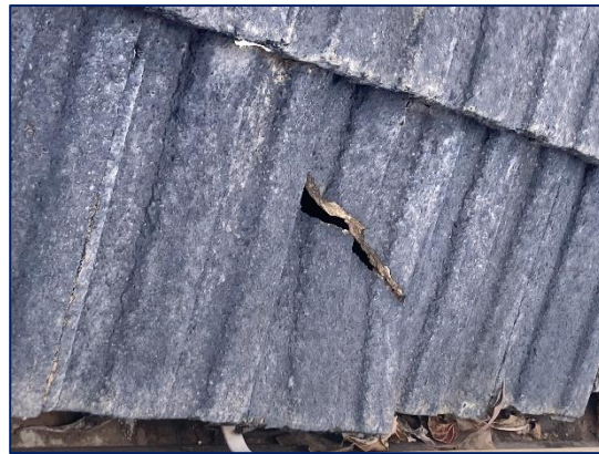
Figure 58: Broken Tile
