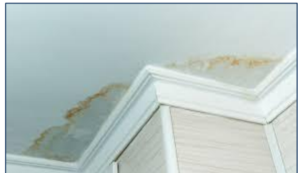
Figure 54: Stained Ceiling
