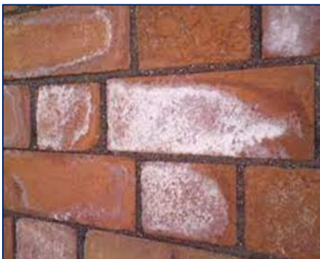
Figure 68: Efflorescence
