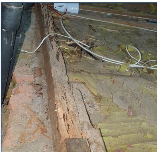
Figure 55: Damaged Rafters
