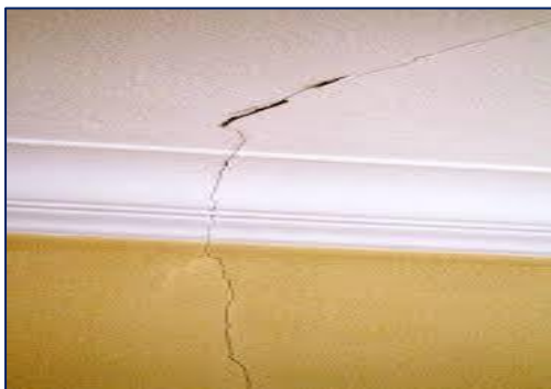
Figure 40: Cracked Ceiling
