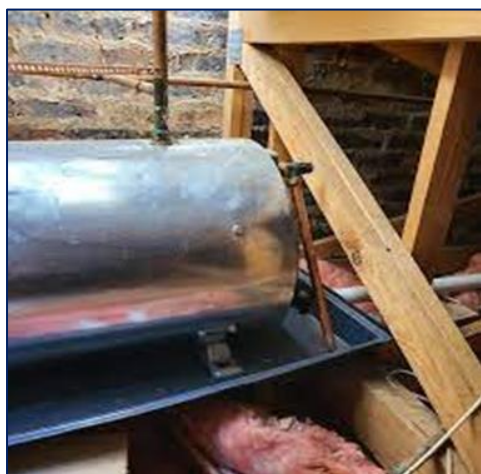
Figure 43: Geyser Drip Tray
