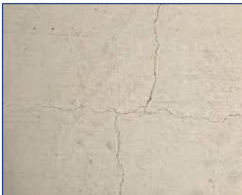
Figure 8: Hairline Cracks
