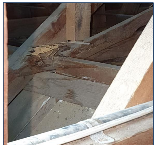
Figure 56: Damaged Trusses
