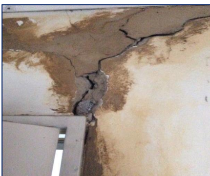
Figure 66: Structural Crack
