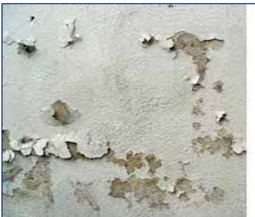
Figure 38: Blistering Paint
